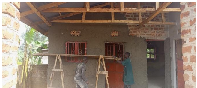
Builder Godfrey and one student working on the plastering
